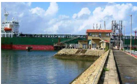
Figure 5: New Kipevu Oil Jetty, Mombasa.
