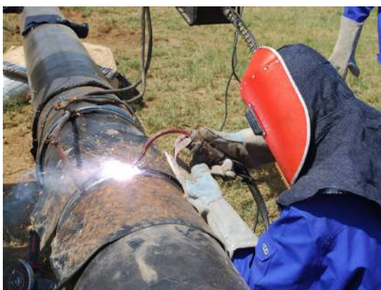
Figure 6: KPC Pipeline Welding and Pumps Maintenance Service
