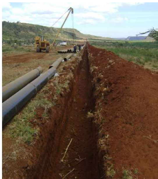
Figure 3: Construction of a 450KM pipeline from Mombasa to Nairobi (Line 5) commissioned in 2018
